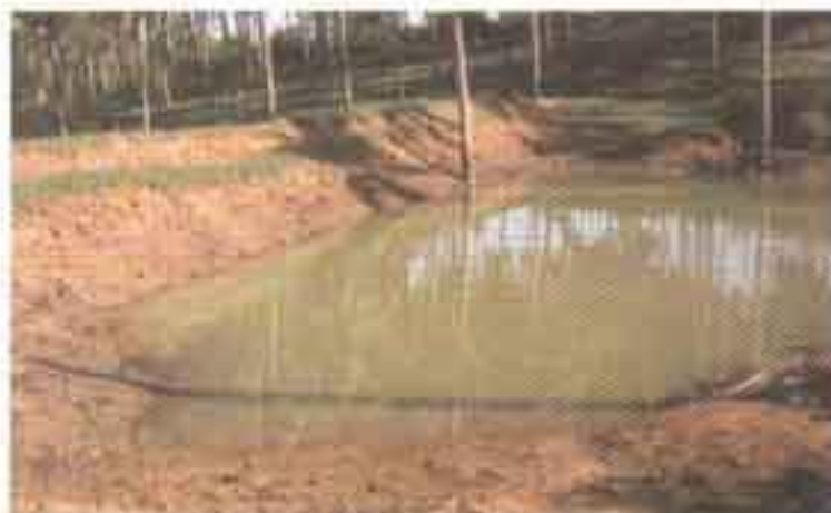
Picture 11: A tank constructed for collecting rain water
