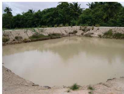
Figure 9: Rain water harvesting tank
